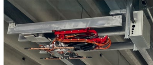
Overhead pantograph at Shepherd Parkway
